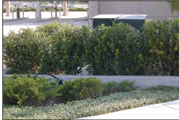
Illustration 5-10 LANDSCAPING ELEMENTS DO NOT PROVIDE ADEQUATE SCREENING IN THIS EXAMPLE
