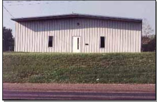
Illustration 5-12 THE “VIEW FROM THE ROAD” OF A METAL BUILDING
